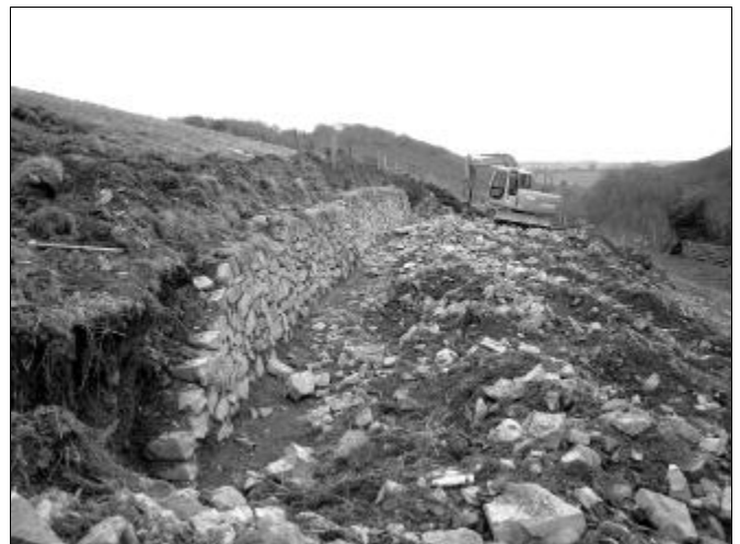
The creation of the stone bank in Forde Orchard will provide a new habitat for reptiles, insects and plants Photo: Matthew Twigg
